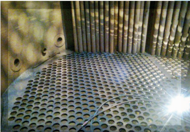
Boiler and Heat Exchanger retubing
