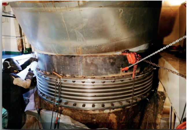
Accommodation Ladder repair and M/E Exhaust gas Compensator Replacement
